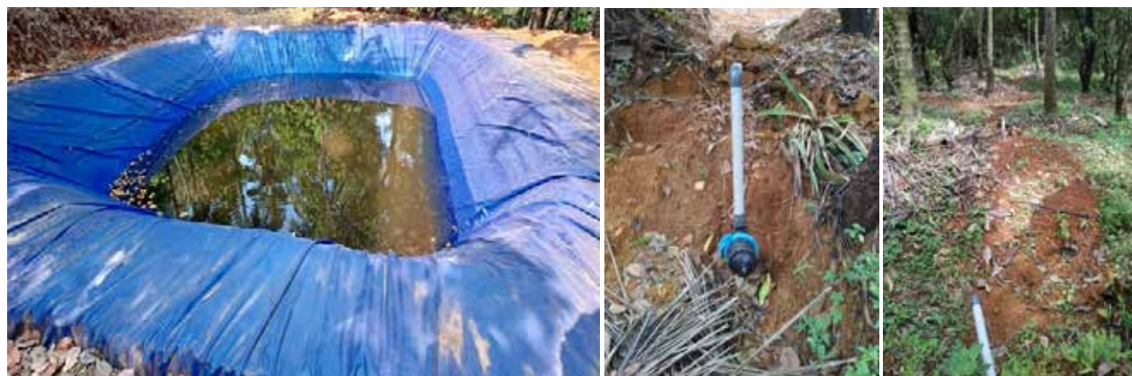
Water harvesting pond with gravity based drip system.
