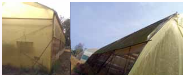
Vertical sides show less algae growth as compared to aerodynamic shape and thus less
