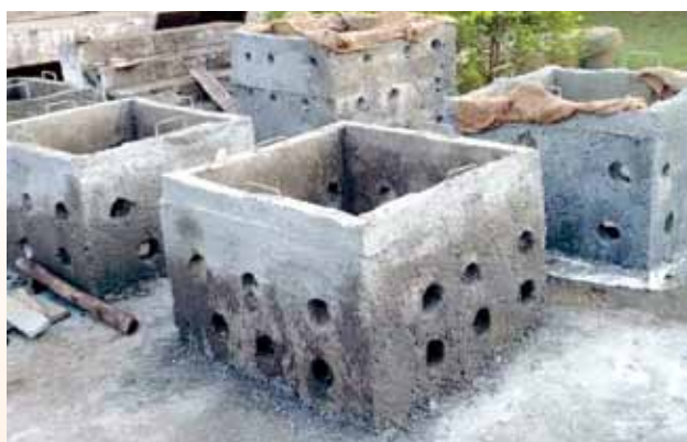
Construction and installation of AFHs
