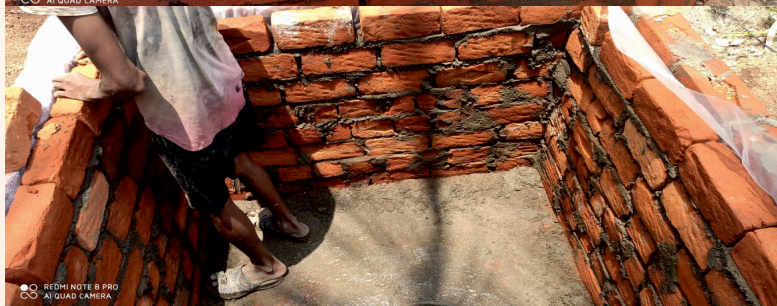
Figure 2: Pusa Bin Cross sectional view Capacity 0.5-4.0 tonnes LXBXH : 610-1720X610-1520X1360-1600 (mm)
